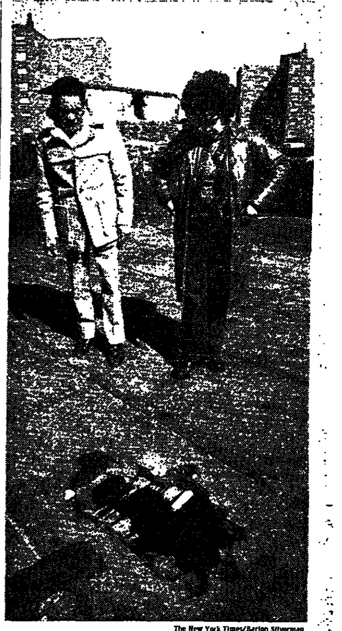
Antonia Fragoza and her father, Carmelo Lacosta, examining a hole in the roof of their apartment house.
